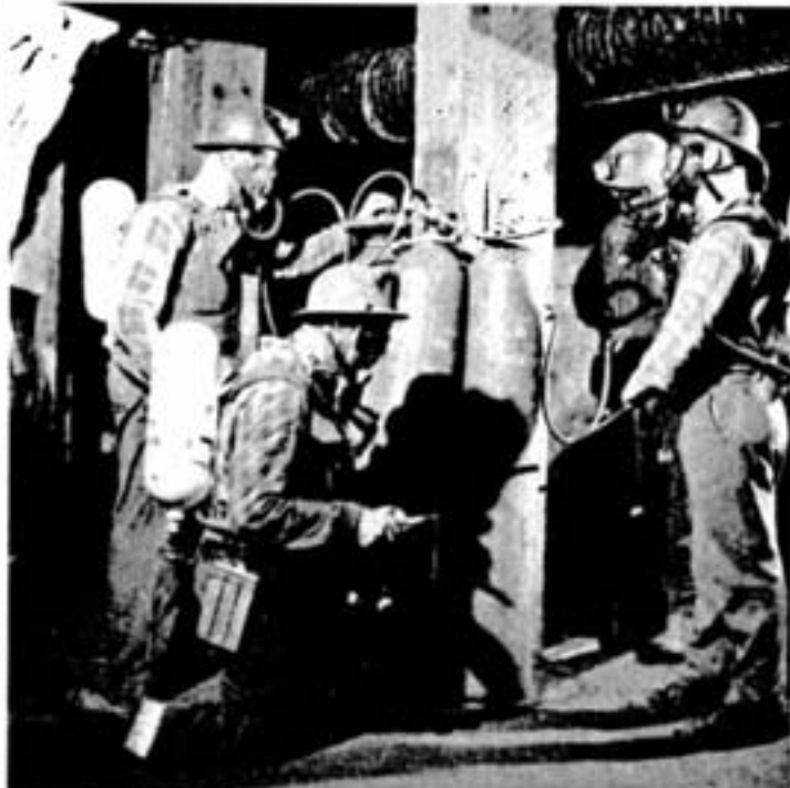
The standard three-bottle cascade system has been set up and is operating here as four mine rescue workers recharge the air bottles on their equipment: Ray Spotton, Ron Witherall, Arnold Sten and John Guthrie.
