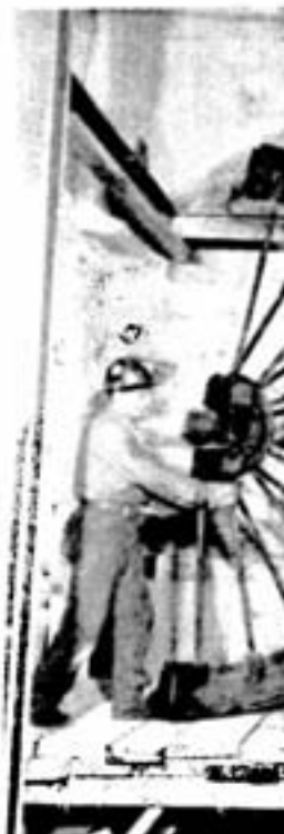
MURRAY: Here we see shaft being hoisted into p above this elevation. Rigger gives signals to hoist ope
