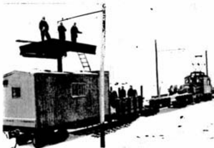
Tightening slack in trolley lines is one of the line car crew's more routine tasks. Note the elevated platform which can be adjusted to the desired height for convenience and which is well insulated for safety.
