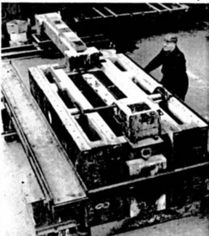
Heaviest copper casting produced at the Copper Refinery is the 11,000-lb. mould made about every six months for the Anaconda Copper Co. at Toronto. This huge block of pure copper, produced to the very high standards for which the Inco refinery is famous, is shown above just after being cast in the foundry. One of the two pouring launders is still in position. Six moulds, held together by massive C clamps, constitute the mother mould in which the Anaconda casting is poured. Looking over the assembly is foundry foreman Henry Limoges.
