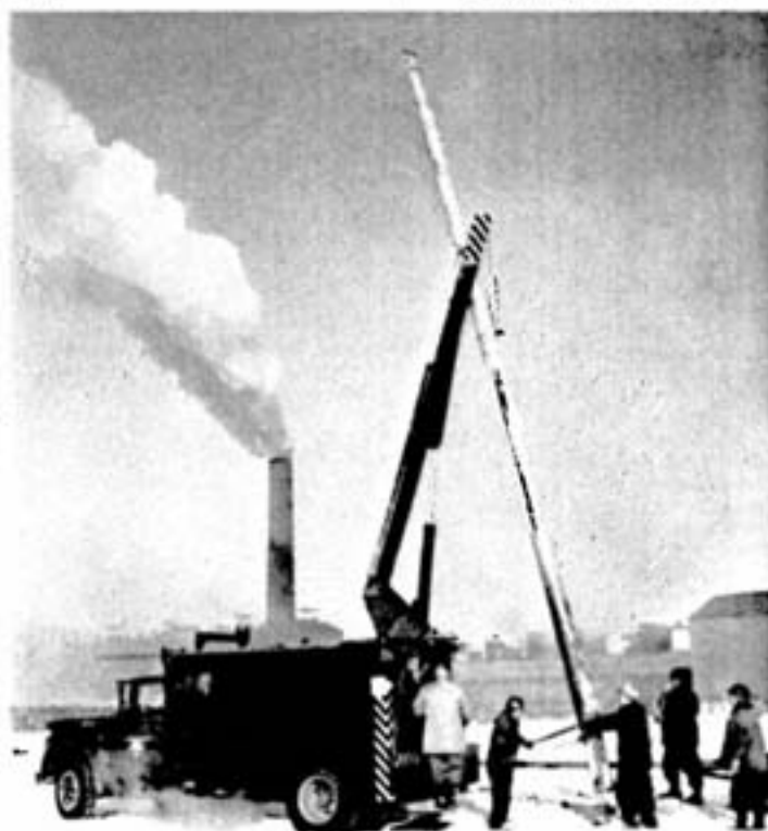
Inco's shining new line truck had its trial run in the smelter yard, setting a standard 35-foot power pole. It performed the job without a hitch, winning the approval of all with its highly efficient hydraulic boom.
