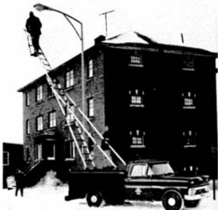
Linemen Bernie Akey and Jack Hunter are seen installing one of the new mercury vapor street light fixtures at Copper Cliff. Installing and servicing street lighting is one of the many services provided by the line gang.
