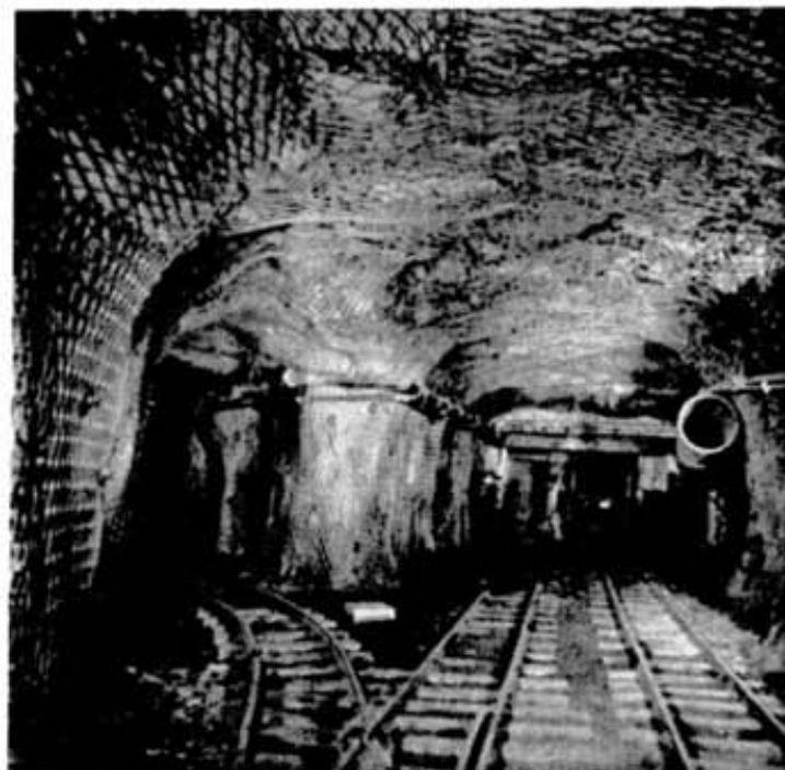
LEFT: A view of the intersection on 6200 level looking back toward the shaft. Here on the left the main crosscut cleaves from the station drift and strikes out for the ore zone. Driller Bernie McDonald selects a steel from the steel rack.
