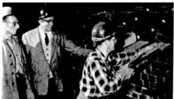
Relining a converter is a big job that uses more than 12,000 refractory brick. Here assistant smelter superintendent Frank Matte checks with mason leader Ugo Rossetto on the progress of a job in no. 15 converter. Roger Sabourin is the mason laying L239A's to brick the back of the converter. Above Roger's head may be seen part of the collar of the converter.
