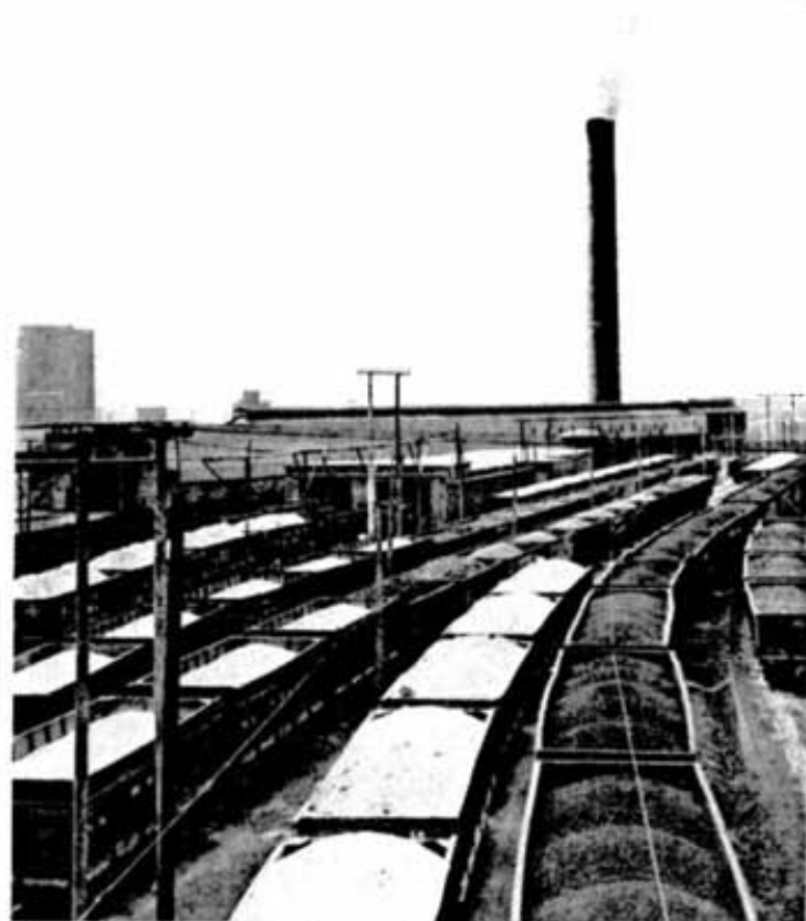
The stock storage area at Copper Cliff shows a variety of furnace feed awaiting disposal. On the extreme left are cars of Levack concentrate, then quartz, converter and magnetic ore, sand and coal.
