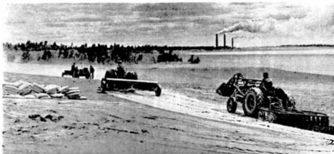
Here is a busy scene at the tailings area west of Copper Cliff as another experimental plot is being prepared for seeding. Lime is being heavily spread and disked in by an agricultural department crew.
