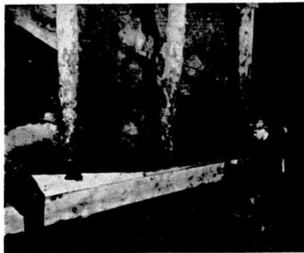
LEFT: Here the ore has been removed and Clarence Young and Alec Duguay are catching up the stringer with a round post in preparation for repeating the mining cycle.
