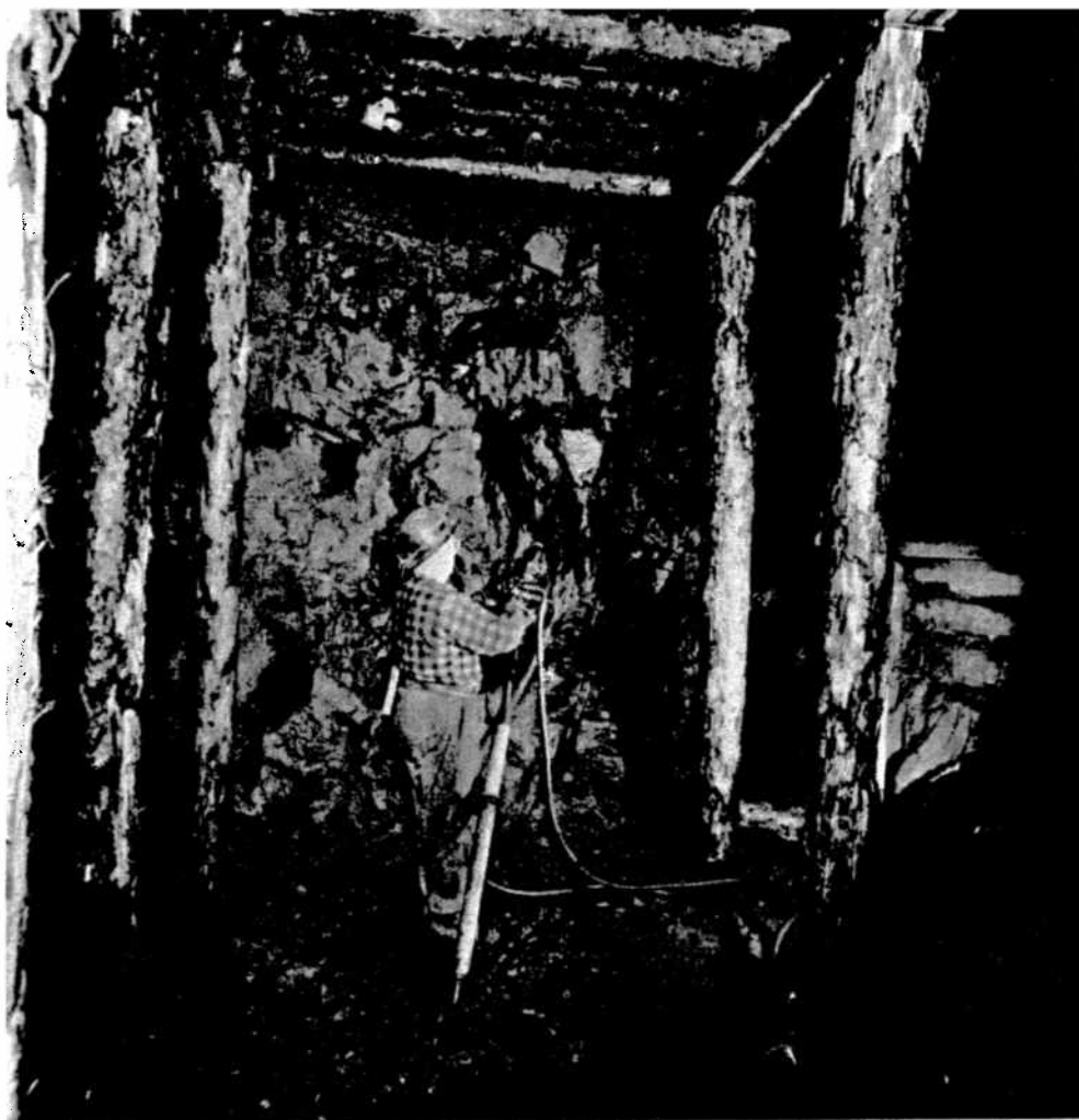
In this view of undercut-and-fill mining at Frood, Leo Dubeau is drilling off a round of holes in the breast. The picture shows clearly the excellent protective overhead cover provided by the mat of logs installed after the previous slice had been mined out.
