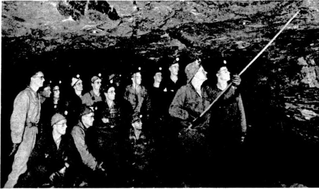
LEVACK: A job demonstration at Levack mine. In 102 stope on Levack's 3000 level shift boss Dave Simpson is seen demonstrating to a group of his men the safe method of scaling. Safety engineer Jim Vettorel may be seen at the left of this group. Demonstrations such as this are another regular feature of the mine safety program.
