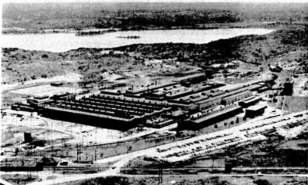
The Inco Copper Refinery at Copper Cliff, shown in this aerial photograph taken early last spring by Michael Dudowich, has some 600,000 square feet under roof, of which about half is occupied by the tankhouse. The first cathodes were pulled in this refinery on June 13, 1930, and the first wire bars were cast the following August 12. Among the important improvements in copper refining practice pioneered here have been direct arc melting of copper cathodes, the transfer of molten blister copper from the smelter using hot metal cars, and the development of machine-pointed vertically cast wire bars. The refinery produces a large variety of regular and special copper shapes for the fabricating industry. In the background of the picture is Kelly Lake.
