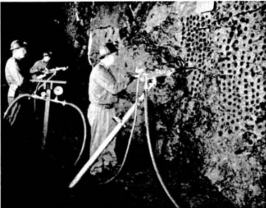
In this view of an underground steel-testing station at Frood-Stobie mine, a drilling crew is conducting a regular test of drill steel. The drillers are Leo Rivest (nearest camera) and Omer Vallee. The test engineer, Fred Horner, controls the air pressures for both machines, and times and measures each run. He also sharpens and gauges the inserts. The picture on the right shows one of the underground drill repair shops which are strategically located in each of the Inco mines; the drill fitter is Al Saulnier.
