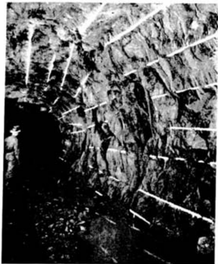
Effectiveness of the shearing action in perimeter blasting is indicated for visibility. The back and wall are cleanly cut, and overbreak reduced right shows the irregular wall and back resulting from conventional
