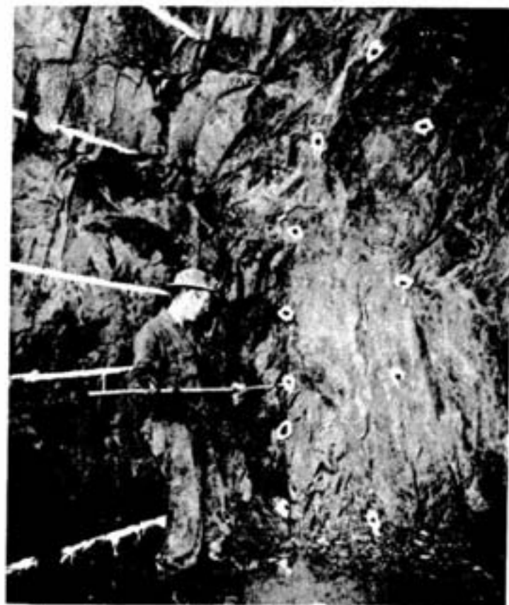
Loading a hole in a perimeter blast in a return air transfer drift at Creighton 3 shaft is Howard Holmes. He shows how cartridges of the new type of powder developed for this blasting technique can be linked to form a continuous train of explosive.
