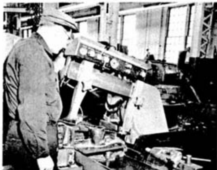
This Do-All hydraulic 12-inch cutoff saw is "Handy as a can opener to a new bride," as Lloyd King put it. Capable of cutting any metal up to 12 inches square or round, it is one of the busiest machines in the shop. Saverio Bussolero is seen splitting a deadeye bearing used in the coal plant.
