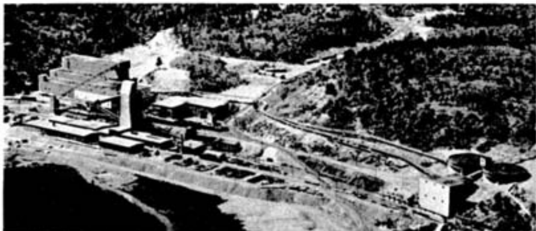
Here is another view showing the close integration of the new 6,000-ton Inco mill at Levack with the mine surface plant. Ore from the No. 2 shaft rockhouse is conveyed directly into the mill's crushing section. Mill tailings are piped 1,500 feet to a sand plant (right) located at No. 1 shaft, where they are used to make sand fill which is sent by pipeline directly into the mine. Rejected slimes from the sand plant are thickened in the two 100-foot Dorr tray thickeners seen in the picture, and are piped to a disposal area.
