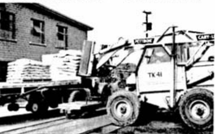
Loading square-set timber onto mine trucks is easy for the fork-lift in this view at Levack. In piling the timber openings are left for the forks of the truck. In the picture on the right a tractor float of cement in pallets is being unloaded at Garson to be taken directly underground.
