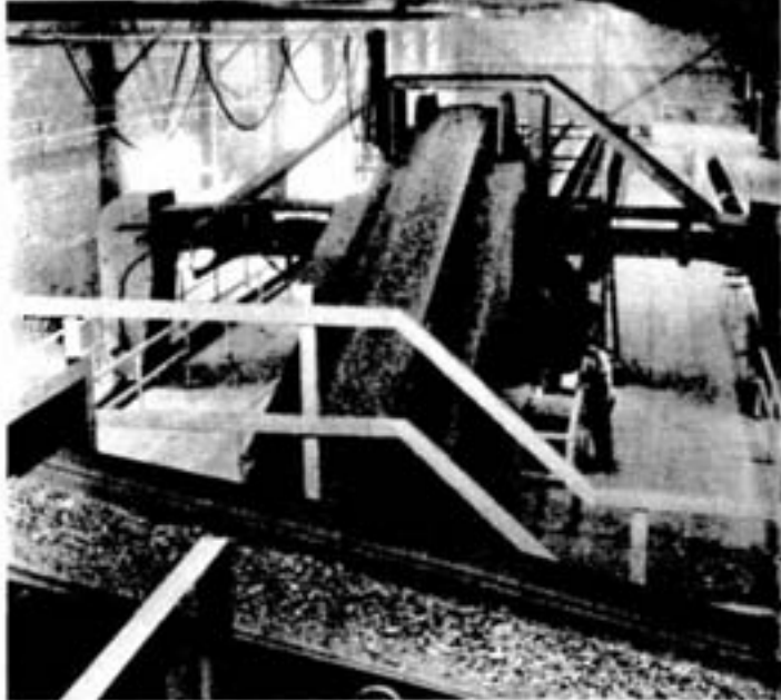
The crushed ore is transferred to the fine ore bins. In the foreground the belts bringing the ore from the crushing section. In the centre of is the tripper which travels back and forth distributing the ore from main conveyor belt through the four long slot openings above the bin
