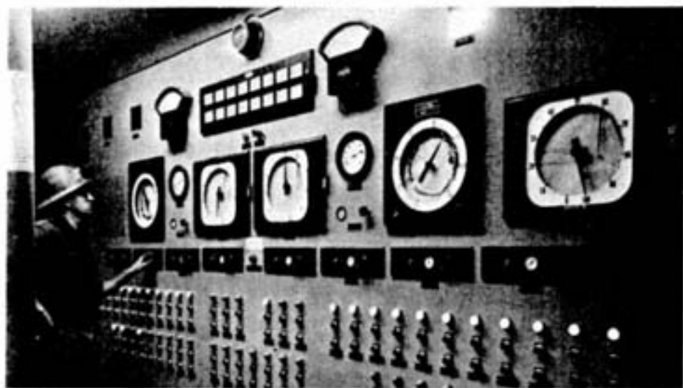
Remote and automatic control has been accomplished to a high degree in the new Levack mill. Here's the elaborate panel for recording and controlling what goes on in the grinding section, from mill feed to pulp density. An alarm is given when trouble occurs at any point in the circuit.
