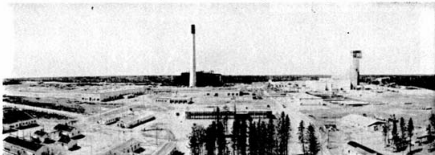
Panoramic view of the plant site area of the Thompson Mine of The International Nickel Company of Canada, Limited, in northern Manitoba. Towering over the smelter construction, in left centre, is the 500-foot chimney, one of the tallest landmarks in western Canada. To the left of the smelter is the permanent shops building. At the right is the concentrator, with the 261-foot headframe of the Thompson Mine 2100-foot production shaft to its right. General office building of the new plant is shown in the centre foreground.
