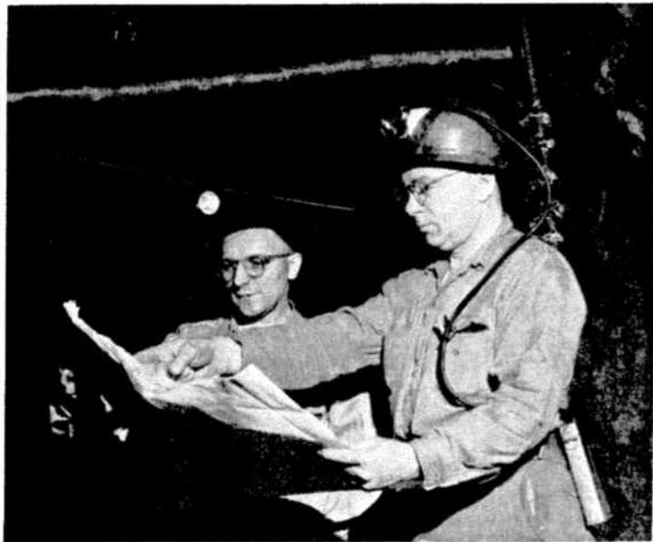
In this picture the division foreman, Walter Sokoloski, is checking the circuit layouts with the assistant layout engineer, Don Obonsawin. Every detail of the blast is carefully planned by the mine engineering department before the operating and electrical departments do their work.
