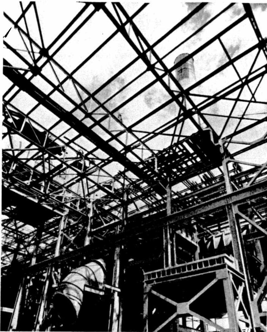
*Reaching for the clouds, the top of the 500-foot chimney is seen here through the skeleton of smelter steel at the International Nickel Company's great new plant at Thompson. Steel workers can be spotted several places in the picture, two of them fixing a block to the top of a flimsy gin pole and others straddling lofty girders with the supreme scorn for height traditional of their trade.*
