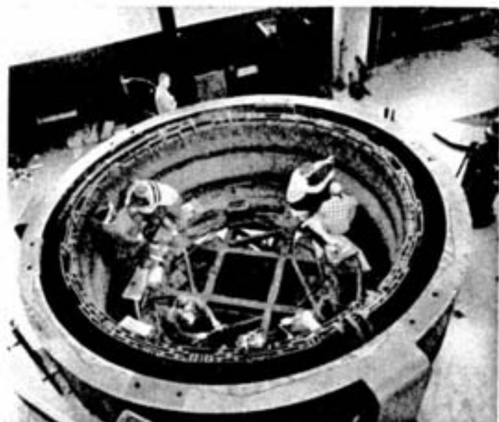
Chick Dunn watches as the rotor shaft is hoisted from inside the stator of one of the three Big Eddy generators, as the major overhaul gets underway. In the picture on the right a group of Inco electricians work swiftly to install the 540 new fibre wedges in the stator coil; they are Bud Germa, Kalevi Hilapiela, Dale Muirhead, Howie Thompson, Hector Steele and Ray Kainulainen.
