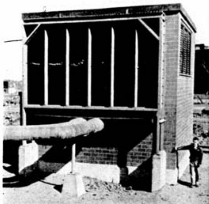
Air Heater The air heater coil, consisting of 840 vertical tubes, is installed in an opening in one wall of the fan house. Openings in two other walls of the fan house allow unheated fresh air to reach the fan during the warmer eight months of the year.
