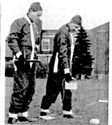
Bill Campbell and Tom Crowther shown as they measured and mapped radiation with a radiac set.
