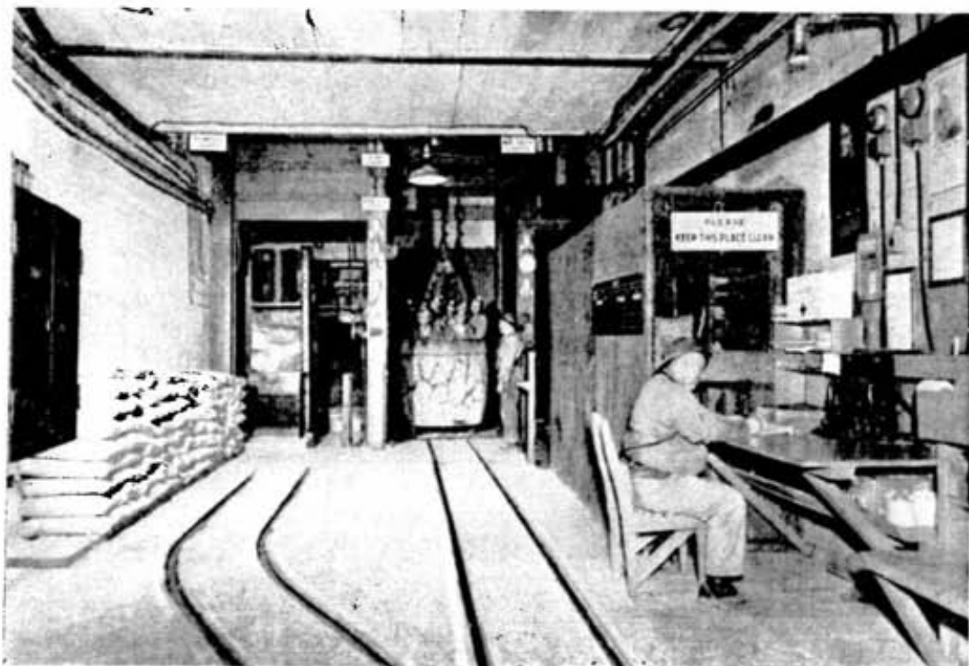
The leader and six shaftmen of a sinking crew have climbed into the bucket and are about to be lowered to the shaft bottom in this view of the "deck" of Creighton's new No. 8 shaft at 64 level. Albert Boucher, the shaft foreman, makes out a requisition at the topman's desk. Bags of cement for shaft concrete are stacked neatly on the left, and immediately beyond them is the measuring hopper into which cement is placed, along with gravel drawn from a bin directly overhead, and then dumped into a concrete mixer installed one set below the level. Standard safety installations for shaft sinking can easily be identified in the picture.
