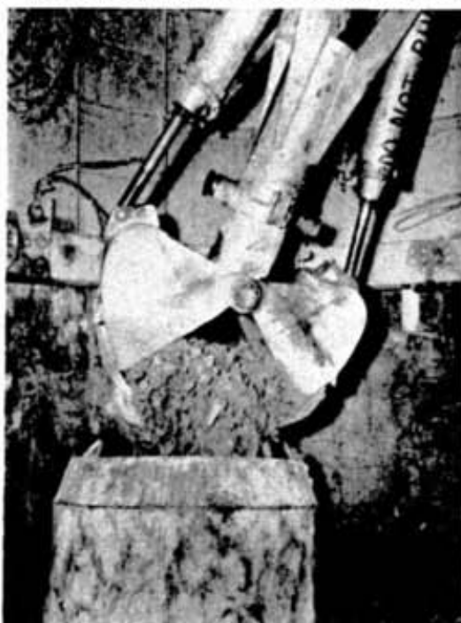
The clam of the Cryderman mucker is seen as it takes a 9-cubic-foot bite from the muck pile in the bottom of the shaft, and then swings over on the end of the boom to drop 400 pounds of rock into the bucket.
