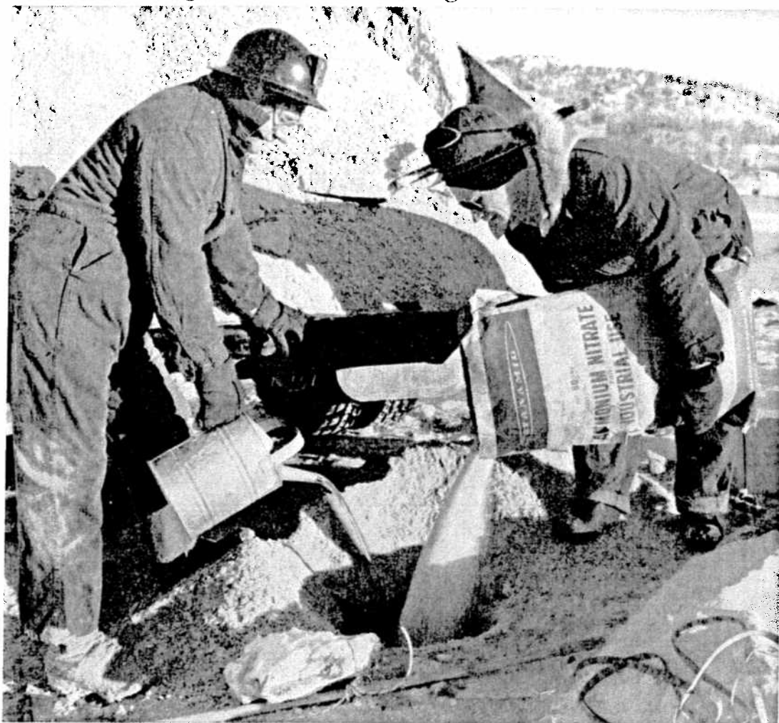
Bill Gibson (right) and his partner, Frank Patterson, blend a blasting charge of ammonium nitrate fertilizer and fuel oil in a churn drill hole at Lawson quarry. The primacord that will be used to trigger the blast is seen in the foreground, attached to a loading stick.
