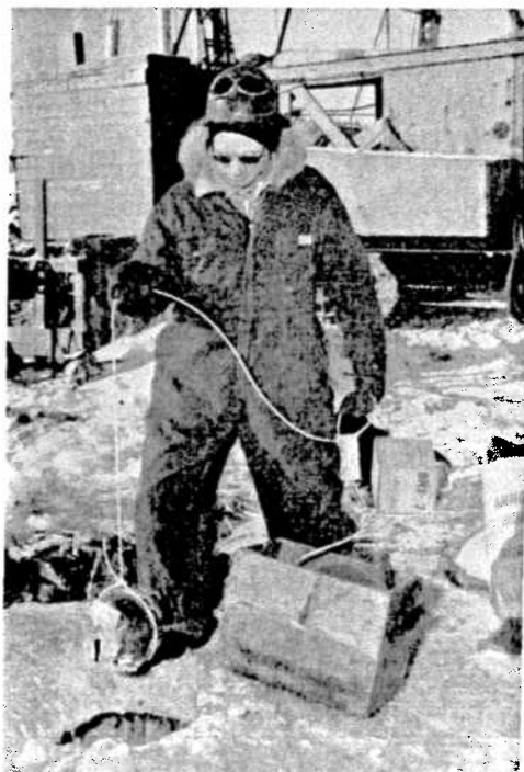
To provide a dry base for the ammonium nitrate, and also to serve as a detonator for this relatively insensitive blasting material, the first few feet of a drill hole is loaded with BRX blasting powder. Bill Gibson is shown on the left, lowering a bag of BRX by means of the primacord detonator. In the centre picture Frank Patterson dumps finely crushed quartz into the hole as spacing between deck loads. On the right Bill Gibson threads the primacord through a pentolite primer, which he was investigating as a possible replacement for BRX in deck charges.
