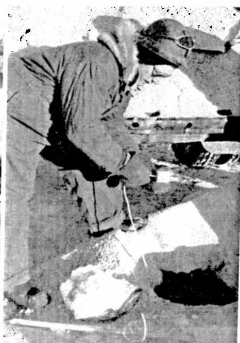
To provide a dry base for the ammonium nitrate, and also to serve as a detonator for this relatively insensitive blasting material, the first few feet of a drill hole is loaded with BRX blasting powder. Bill Gibson is shown on the left, lowering a bag of BRX by means of the primacord detonator. In the centre picture Frank Patterson dumps finely crushed quartz into the hole as spacing between deck loads. On the right Bill Gibson threads the primacord through a pentolite primer, which he was investigating as a possible replacement for BRX in deck charges.
