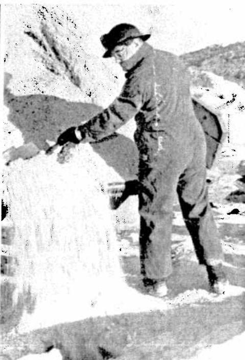
To provide a dry base for the ammonium nitrate, and also to serve as a detonator for this relatively insensitive blasting material, the first few feet of a drill hole is loaded with BRX blasting powder. Bill Gibson is shown on the left, lowering a bag of BRX by means of the primacord detonator. In the centre picture Frank Patterson dumps finely crushed quartz into the hole as spacing between deck loads. On the right Bill Gibson threads the primacord through a pentolite primer, which he was investigating as a possible replacement for BRX in deck charges.
