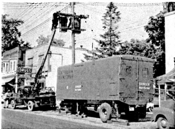
This photograph illustrates the mobility of the Hydro changeover. In the big van is a 100 kw. frequency changer which temporarily supplies 60-cycle power to an area while workmen switch the lines from 25 to 60 cycle.
