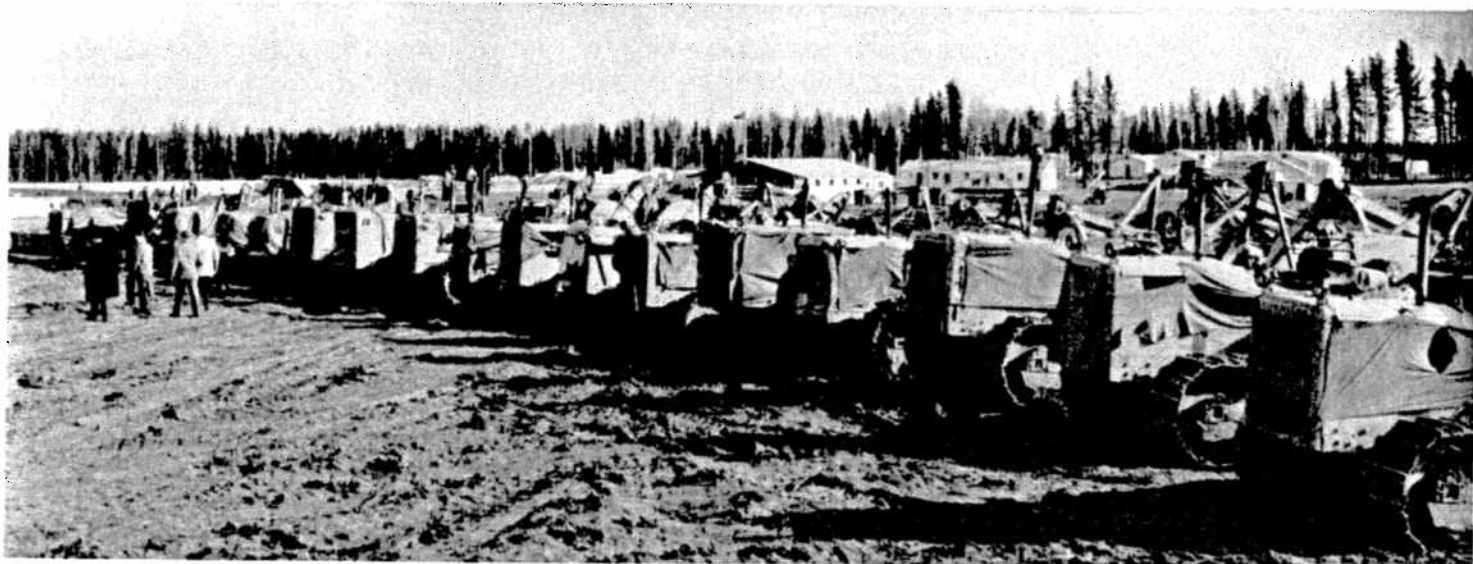
This is the fleet of powerful earth-moving equipment used by Foundation Company of Canada to clear the site of the mill and smelter at Inco's nickel development at Thompson, in northern Manitoba. In some spots of the plant area as much as 18 feet of clay overburden had to be removed to uncover bed rock on which to build the foundations.
