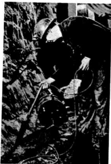
George Fleming prepares to lower the transmitter coil in a "lost" diamond drill hole.
