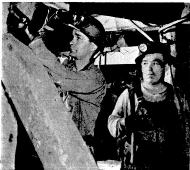
A pillar leader at Creighton mine, where he has been employed steadily since 1946, Archie is seen here at work in 45.1 pillar on 46 level of No. 5 shaft, installing an angle brace with the help of his partner, Julien
