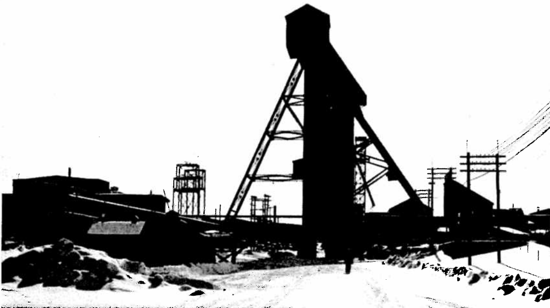
Silhouetted against the winter sky here are the headframe and surface buildings of that grand old veteran of Inco mining operations, Creighton No. 3 shaft, which now fills a new role in its illustrious career. It is the supply shaft handling men and materials for the Creighton caving mining program, the ore from which is hoisted in No. 7 shaft.
