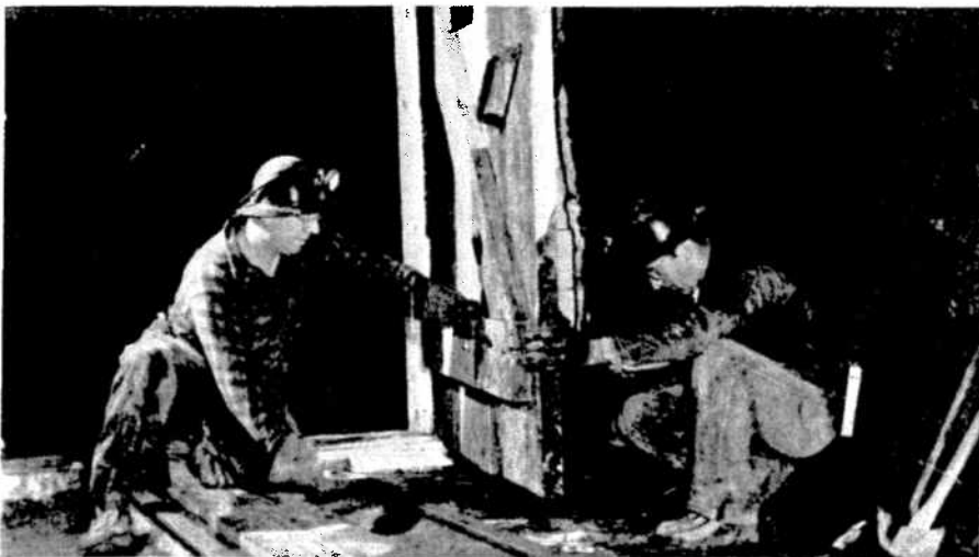
Trimming the bottom of a ventilation door to make a snugger fit, in this picture taken on Creighton mine's 20 level, are George Syvokas and Bill Lucky.
