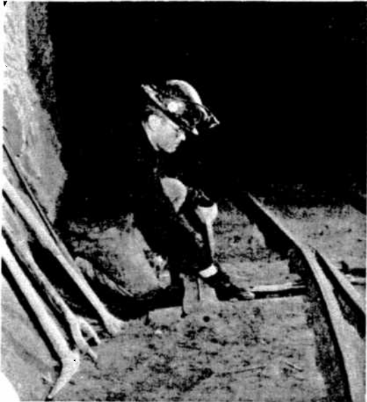
Replacing the bolt holding the throw to a switch bar is a Creighton trackman, Radojko Dobrik.
