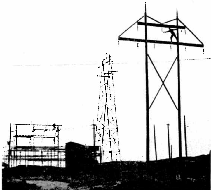
Standing on the cross-arm of one set of poles of the new line that will soon deliver high voltage power directly to the copper refinery instead of via the Copper Cliff substation, lineman Peter Stos connects the wires to the insulators.
