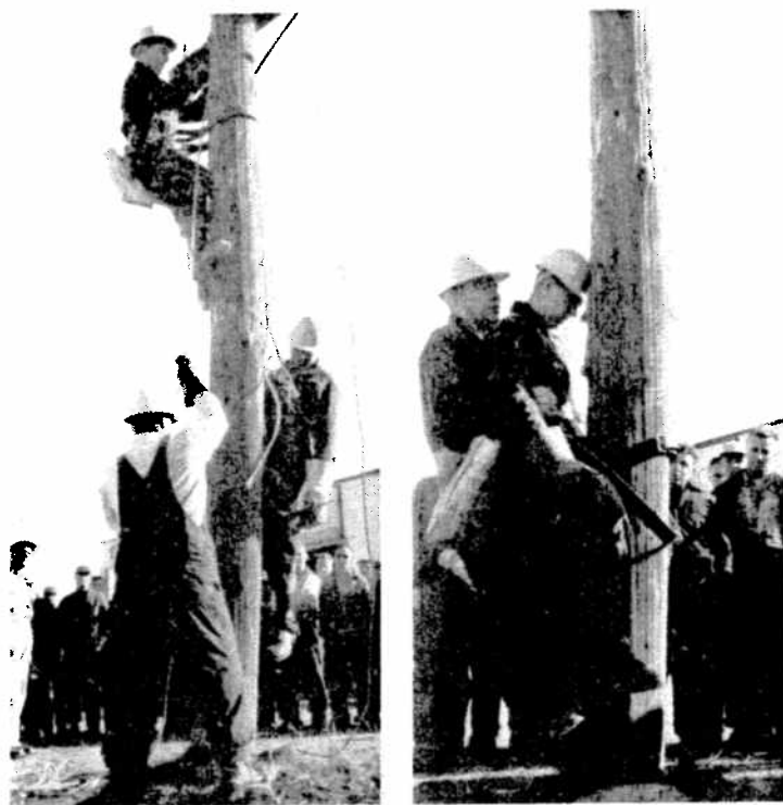
Field engineers of the Electrical Employers' Association demonstrate two phases of rescue work for line crews. On the left two men are lowering an injured workmate from a pole, and on the right pole top resuscitation is being carried out.
