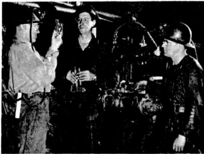
Don Meredith, Garson mine geologist, reads an acid test to check the inclination of drill hole with Leo Dufour, drill foreman, and Dorice Pelletier, driller.
