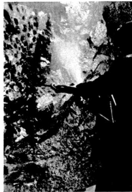
In the steel testing station at Frood-Stobie No. 7 shaft Vic Freelandt is seen as he maintains an even air pressure of 85 p.s.i. on the drill operated by Mickey Banks and keeps a performance record of the steel being used. The broad white line down the breast is the dividing line between two of the six panels in the station. At the right are shown some of the hundreds of holes drilled with various types of steel submitted by the manufacturers for testing.
