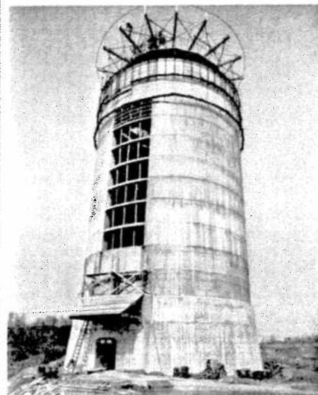
The $19,000,000 plant has taken less than two years to build. Picture shows the 637-foot chimney in an early stage of construction.
