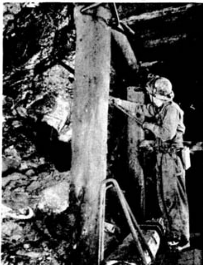
Omer Bedard is scaling the back in a square-set stope at Garson. Note that he is completely covered by the timber overhead, and his feet are protected by the bulkhead. The area behind and beside him is clean. He has a good straight bar, a well-balanced stance, proper foot protection, and glass goggles.
