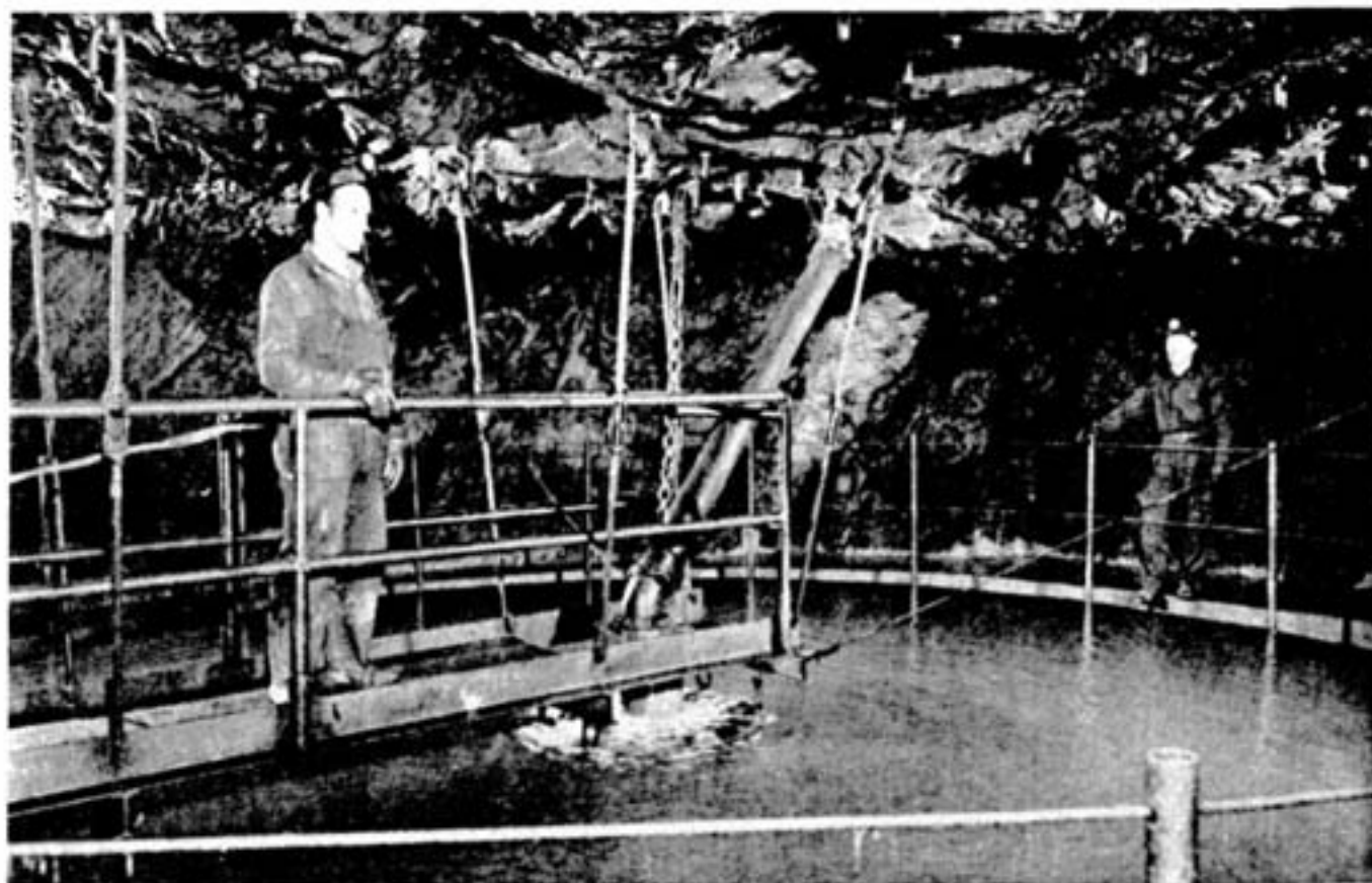
J. Lemieux stands on the cone settler's platform, from which he can adjust or repair the distributor box in which are installed four vanes to break the rush of the incoming mine water. At the right is A. Woschda.
