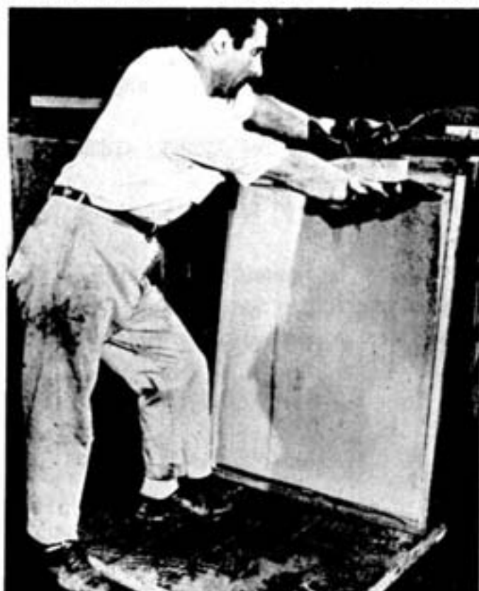
Donato Deluca, in the first of the above pictures, strips a sheet of cobalt from the stainless steel blank on which it has been electrolytically deposited at Inco's Port Colborne Refinery. In the second picture some of the first shipment of electrolytic cobalt from the Port Colborne Refinery is being inspected by R. C. McQuire, manager of Inco's Nickel Refining Division.
