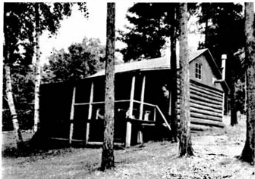
A closeup of one of the four attractive housekeeping cabins at the Coones camp. Percy dragged the logs out of the bush, flattened them on one side with a broadaxe.
