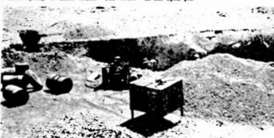
Air for the drills was supplied from the portable Ford V-8 engine at the edge of the pit, four pistons being used for power and the other four for compressing air.
