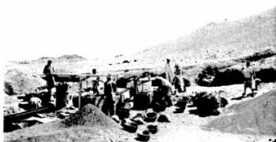
A general view of the concentrator, with the open pit in the background. Baskets were used to carry the ore from the pit to the trommels and then to the concentrator.
