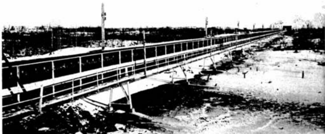
The three-stage conveyor at Creighton carrying ore from the rockhouse at No. 5 Shaft to the concentrator is 1,461 feet long.
