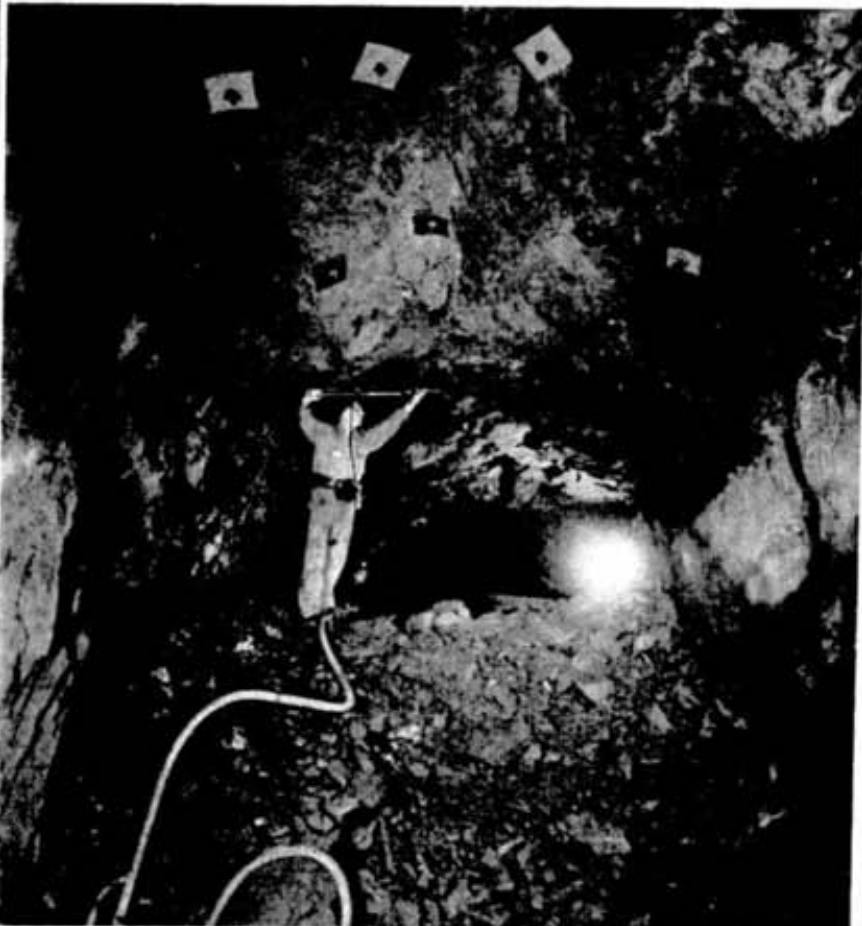
This is an example of roof bolting in a standard Garson drift which otherwise would have had to be timbered. Testing bolts with a torque wrench is Foreman Ralph Armstrong.
