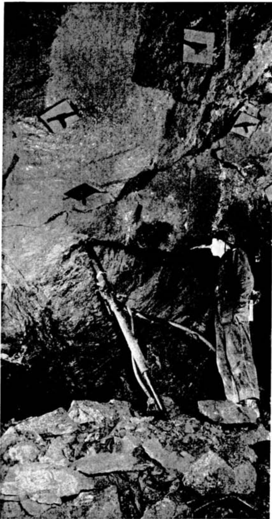
In a cut-and-fill stope at Garson Mine, Paul Korchouski, stope boss, is operating a stoper to drive a roof bolt tight on its wedge. Several roof bolts are seen in place in the back, or roof, of the stope. Six feet long and firmly anchored, they lock the ground tightly into a self-supporting arch which requires no timber.
