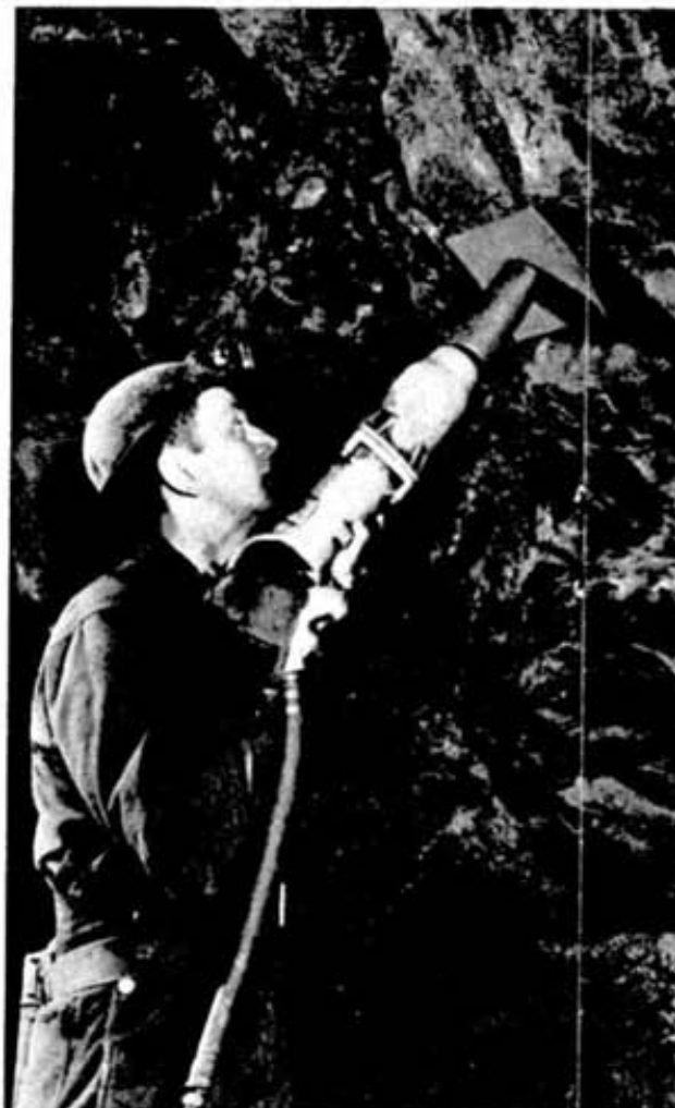
Shift boss Jack Ferguson demonstrates how a roof bolt is tightened to a tension of 7 tons with an impact wrench.
