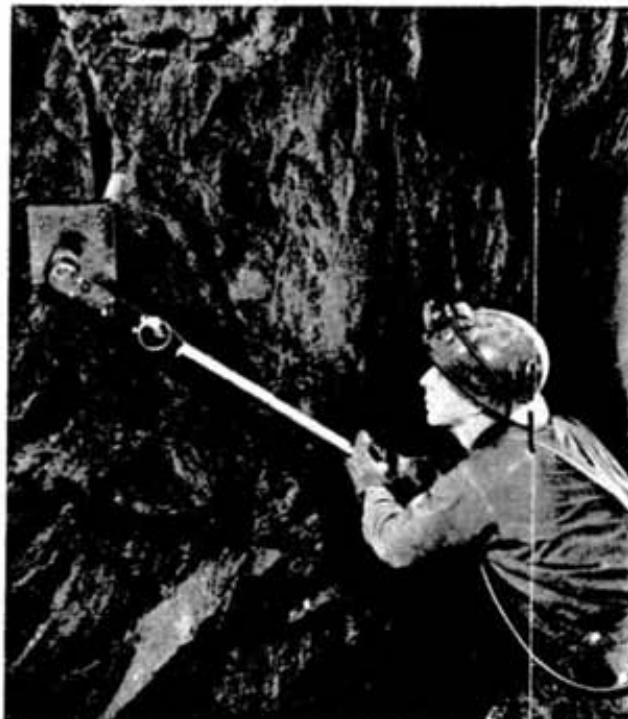
Here Jack Ferguson uses a torque wrench to check the installed tension of a roof bolt. Spot checks such as this, and further periodical inspection of roof bolts with a hydraulic pull tester, are a regular assignment for mine supervision.
