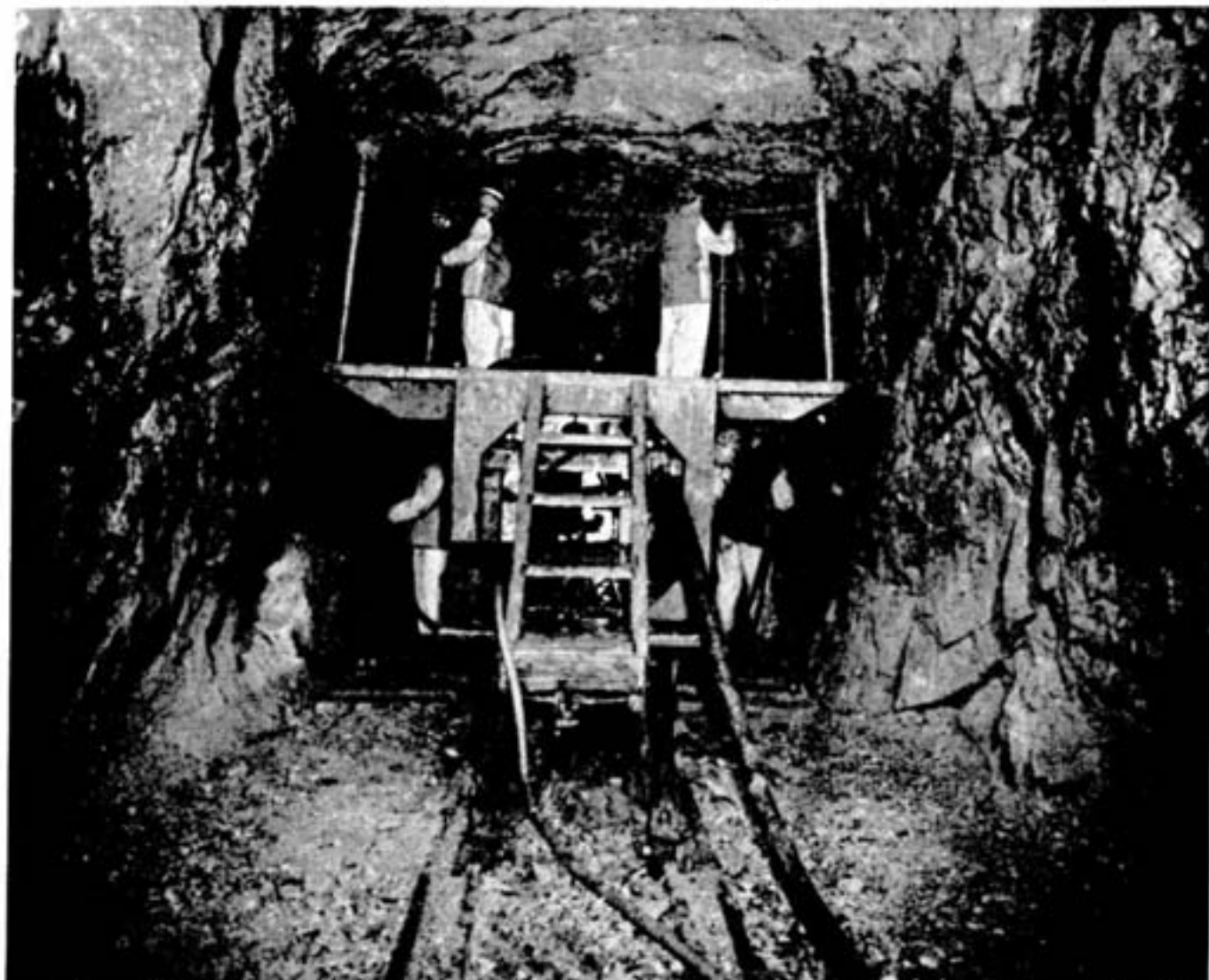
Five air leg drills are operated simultaneously in the high-speed drive to complete a main haulage way between No. 2 and No. 3 Shafts on 2,650 level at Levack Mine. The special drill carriage, designed and built by Inco's mines department for the operation, folds up for convenient removal during blasting. Four of the drillers can be seen clearly in the above picture; the fifth is almost completely hidden by the drill carriage.
