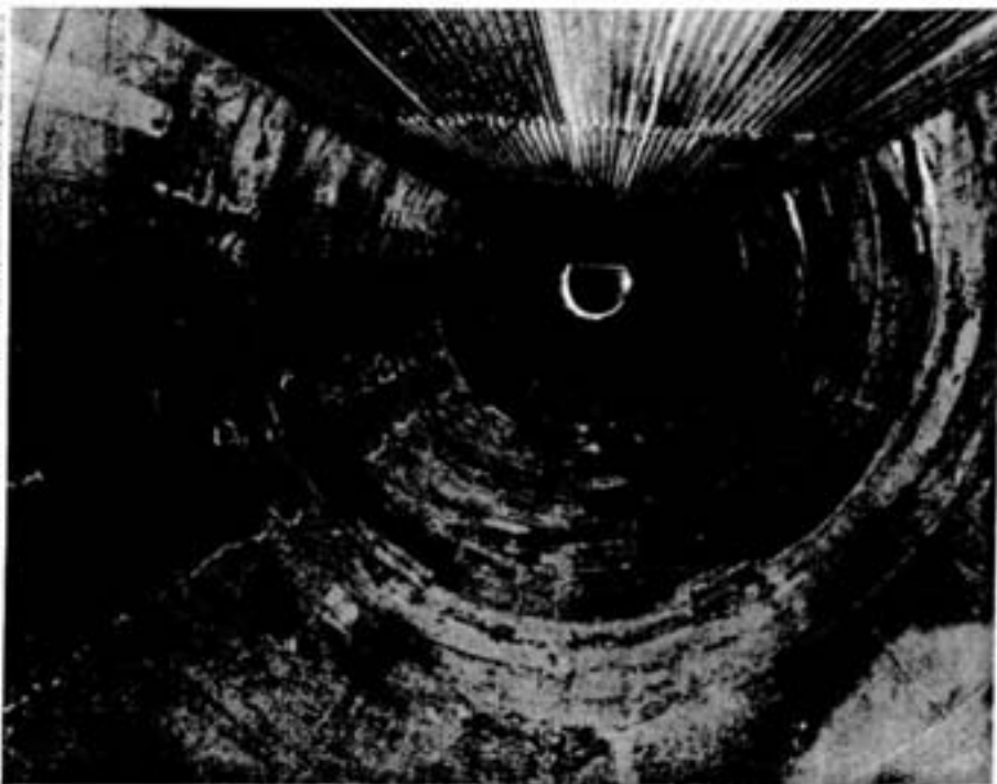
Looking up this 200-foot section of finished airway, from 60 to 58 levels, can be seen two of the eye bolts which supported working platform at one stage in construction.
