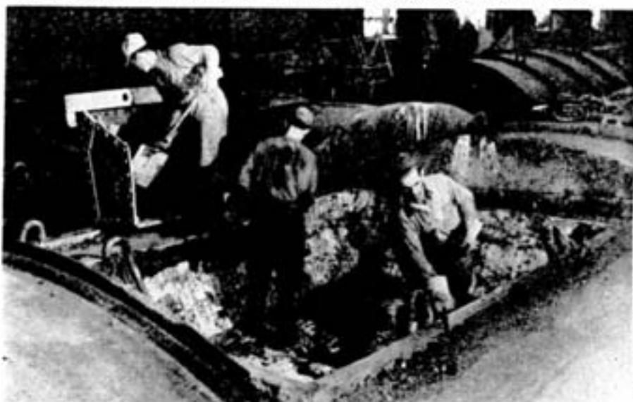
Swamp clay is being used here to streamline a matte mould. E. Belanger (nearest camera) and V. De Grechie apply the clay, J. Beausoleil shovels it from the box.
