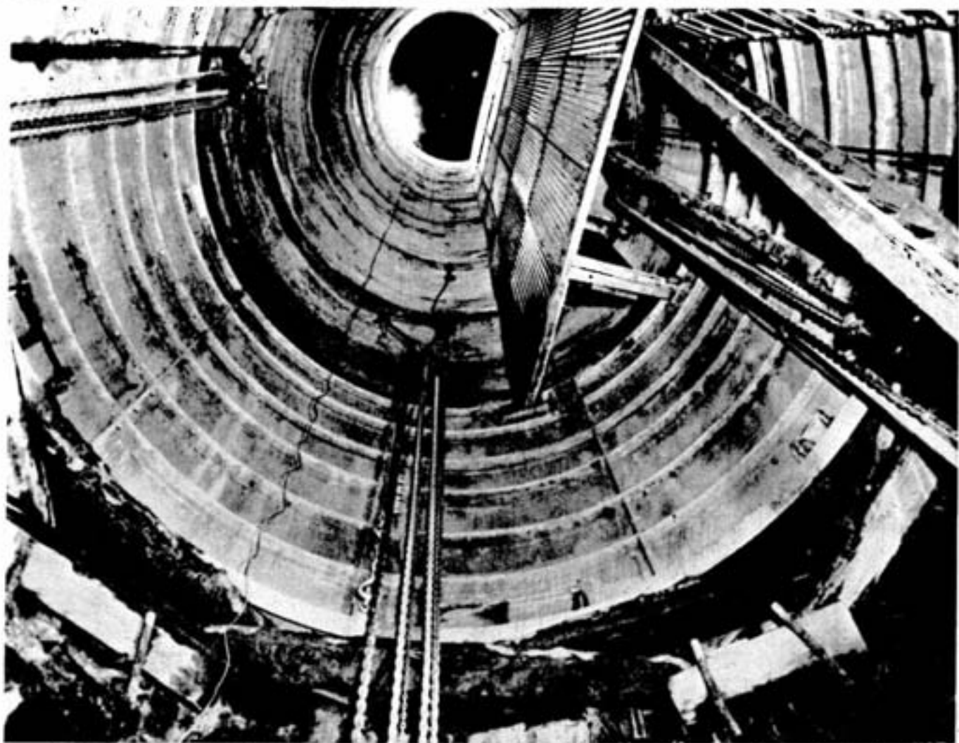
Part of the sectional steel forms are seen in place, supported on pins and blocking, ready for pour of concrete. Also in picture are manway compartment partition, manway ladder, concrete pour pipe, and three of four platform chain blocks.
