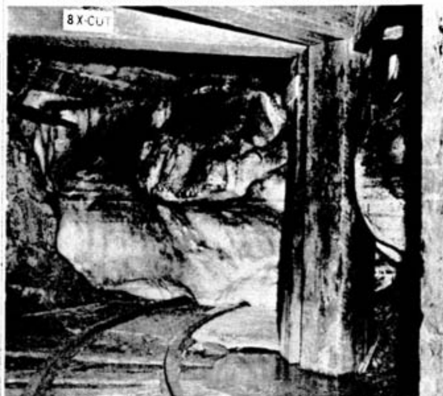
At Creighton they sometimes have to mine ice instead of ore. In the old workings at No. 3 Shaft the down draft of cold air during many winters has frozen seepage water and filled some of the drifts solid with ice. When openings such as the old crosscut shown above are required in the new caving program, the ice has to be mined out with picks or streams of water. Some old boxholes were reopened by mining with heat—melting the ice with big electric elements and fans.
