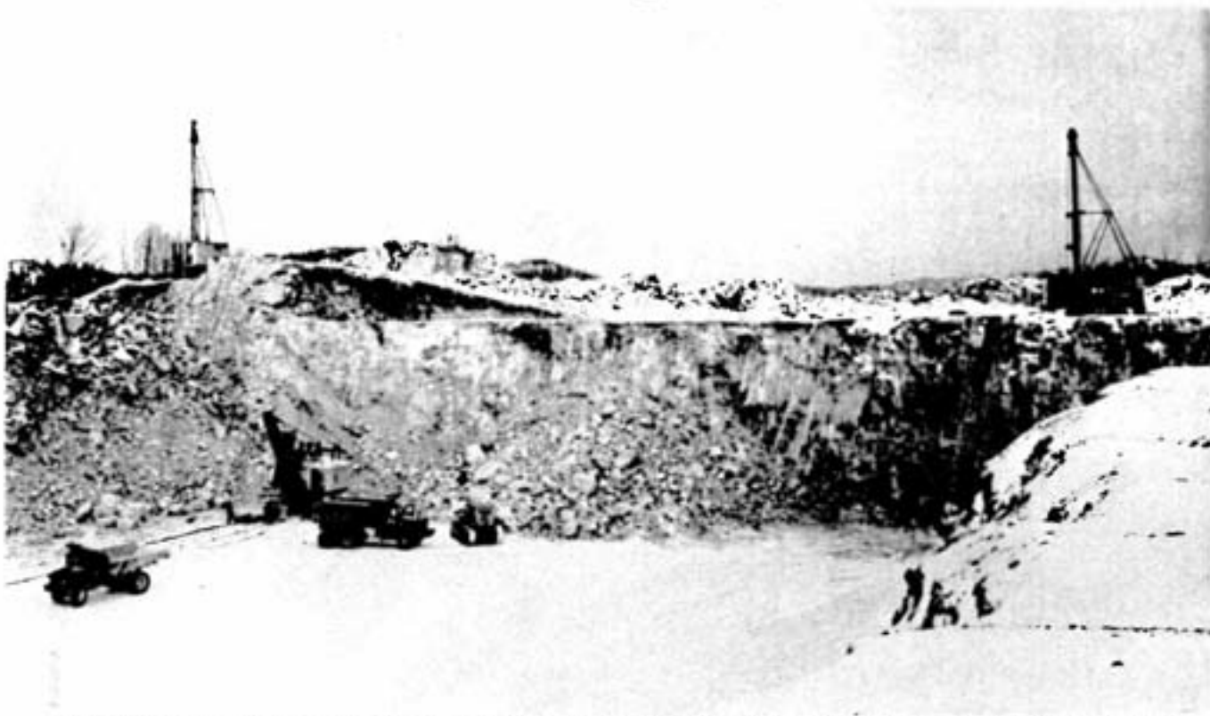
Lawson Quarry, near Willisville on the road to Manitoulin Island, can be a pretty chilly place on a winter's day; you can almost feel the bite of the wind as you look at this photograph. In the pit an electric shovel is preparing to load one of the big haulage trucks with quartz which will be hauled to the crushing plant for processing and then shipped by rail to Copper Cliff for use as flux in the smelter converters. From the top of the bank rise the masts of two churn drills.
