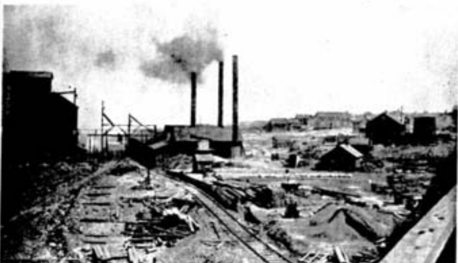
Taken about 1901, this historic print shows the rockhouse of No. 2 Mine and the old West Smelter at Copper Cliff, situated just about where the Oxygen Plant stands today. Rising behind the rockhouse is a cloud of sulphur smoke from the roast beds, which were later moved to O'Donnell. The loading platform in the foreground, and a few of the houses, still stand.
