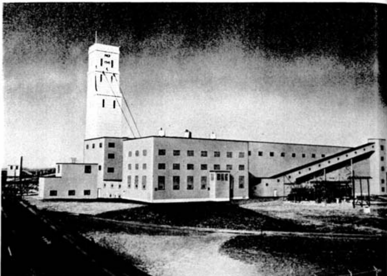
Concrete headframe of the new No. 7 Shaft and the new 10,000-ton concentrator at International Nickel Company's Creighton Mine, seen above, went into operation this year. The $17,000,000 Creighton project is part of a program to boost the annual hoisting capacity of Inco's five underground mines in the Sudbury District to 13,000,000 tons per year, compared with 5,700,000 tons of underground ore hoisted in 1950. The complete program has already involved capital expenditures of more than $100,000,000. Pipeline in the left foreground carries bulk concentrate from the Creighton mill to the Company's reduction plants at Copper Cliff, a distance of seven miles.
