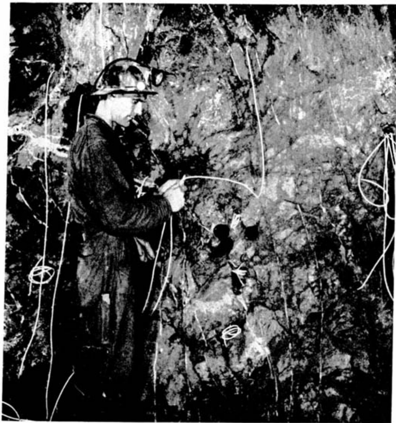
Trimming Fuse Prior to Blasting, Garson
