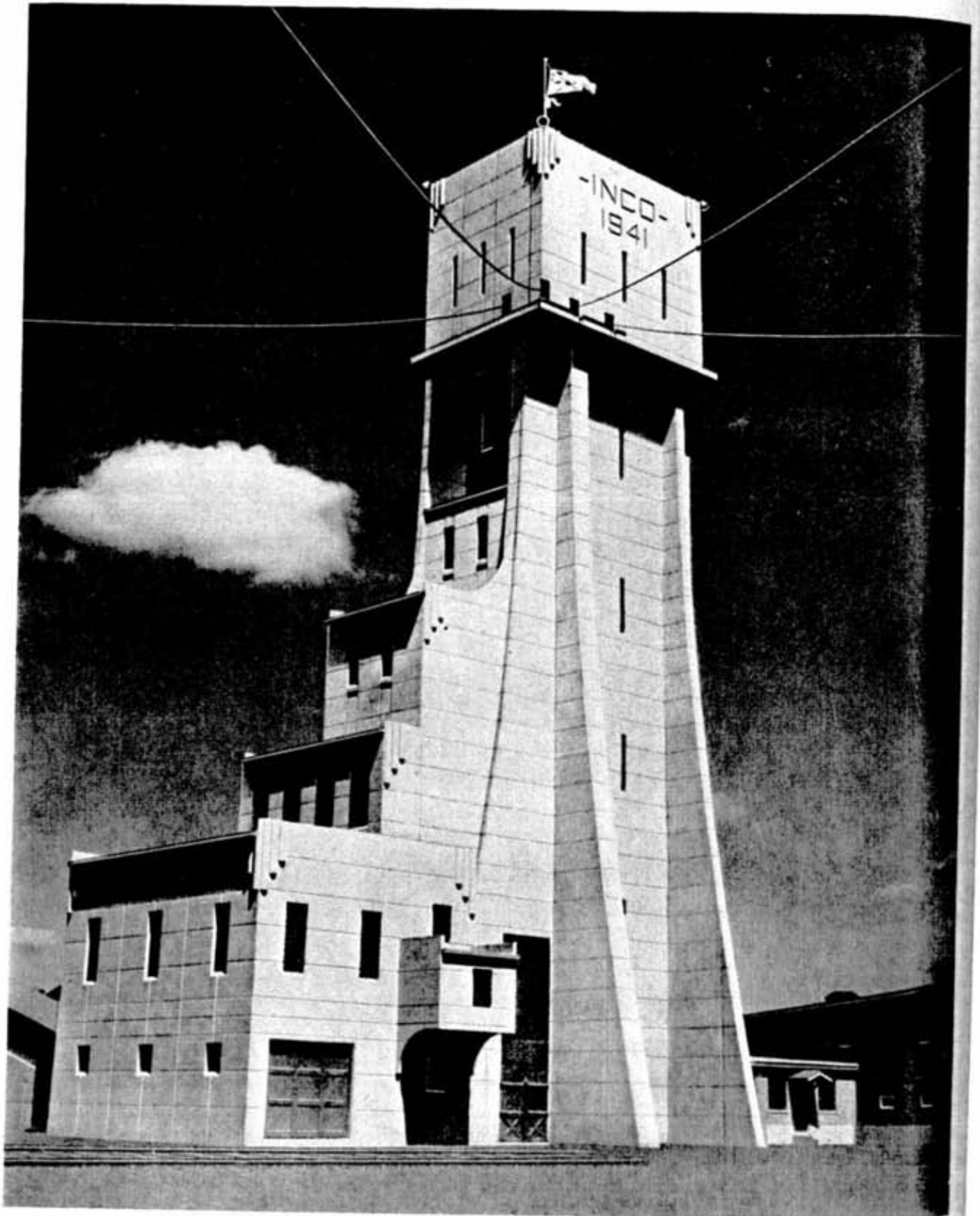
Tugging at its mast atop the beautiful monolithic headframe at Murray Mine, a Victory Loan flag symbolizes the triumph of INCO employees over a high quota assignment in the Sixth Loan Campaign.
