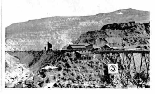
several properties. Prominent were the Chino Copper Co., in New Mexico, and the Phelps Dodge Co., at Ajo, Arizona. The photograph represents the open pit at Chino. This is a typical pit operation. By that is meant the ore body lies below the level of the surrounding country and it is necessary to run spiral tracks along the benches on the sides of the pit. On a pit operation the trains go down into the pit empty and come back loaded.
