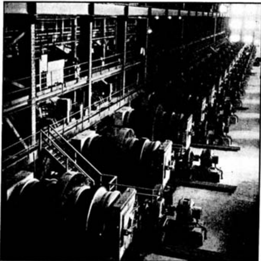
The battery of 17 rod mills in Copper Cliff concentrator, where metallurgy does with ore what surgery can't do with people, and separates the "Siamese twins." A novel experiment is being tried on one of these big mills, whereby it broadcasts its own appetite. A microphone is placed beside the mill, and if insufficient feed is passing into the machine the louder rolling and rumbling of the rods is picked up by the "mike" and passed to a relay, which automatically increases the amount of feed. On the other hand, if the mill is getting too much feed, the consequently heavier slush inside will deaden the normal sound of the rods and then the "mike" passes on the message to cut down on the ore calories and vitamins.
