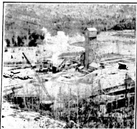
A busy construction scene is the new No. 2 Shaft at Levack. In the centre is the temporary headframe, below which Steve Yawney and his men are sinking the new shaft. Behind the headframe the changehouse and offices are under construction, and in the right foreground the new hoisthouse is being built.
