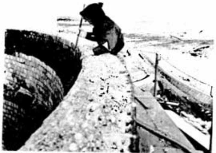
Bundled up in a winter coat to protect himself against the frigid winds 400 feet above the ground, this fellow pries apart the stack's brick lining. Immediately behind and below, the roof of the Copper Cliff mill can be seen. To the right, in the distance, are the white buildings of the Clarabelle mill.
