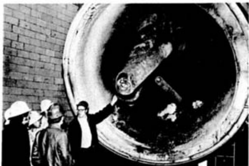
"This is a process lance and fume duct hood belonging to one of our converters," a Copper Cliff nickel refinery guide tells his visitors.
