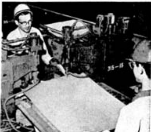
Here's a closeup of a spot-welding machine. One operator positions the starting sheet while the other (facing camera) spotwelds the two nickel suspension loops to the end of the sheet. The operators shown are Paul Havelland and Earl Dadd.
