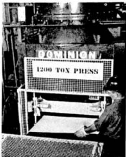
In the hydraulic press the INCO trademark is imprinted in the starting sheet which, when it has grown to a full cathode, will still clearly show this symbol. The press also imprints lines from corner to corner of the starting sheet to stiffen it. Shown feeding a sheet to the press is Les Hanson.
