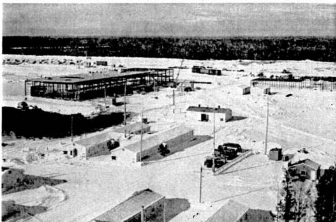
The steel framework of the permanent shops building (left) and the warehouse are seen in this late-winter photograph of the Thompson plant-site area of Inco's new nickel mining project in northern Manitoba. Housing for construction workers is seen in the foreground. The project is scheduled for an annual output of 75,000,000 pounds of nickel by 1961.
