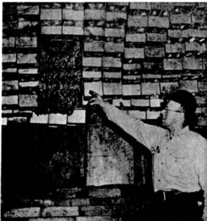
Inside a reverb furnace Henry Beauchamp points to the contrast between new roof cans and those which are partly fused and coated with furnace feed after being in service for two or three weeks. The picture also shows how the cans are stepped down to form the shoulder of the furnace roof. Below the shoulder can be seen some of the big sidewall cans.
