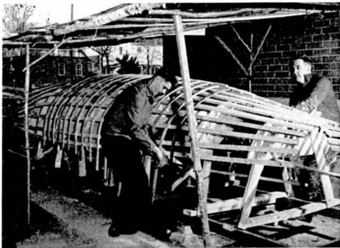
"Easy does it" says Gerry Smith to son Ken as they bend another oak rib in place on the sailing sloop they are building. If not handled with care the ribs crack. The pine battens that shape the boat are seen running lengthwise over the form boards. This is the first boat Gerry has built.
