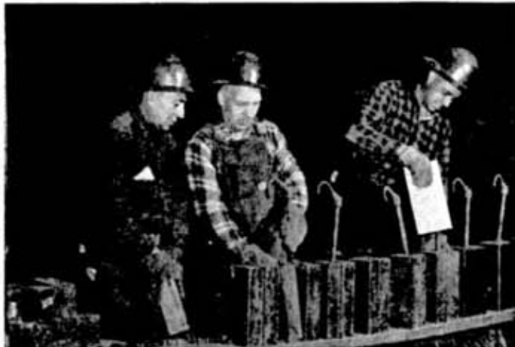
In the brick shed "Blackie" Tarricani, Ernie Levesque, and Jim Ross are assembling roof cans, which consist of two magnesite brick, a steel spacer and container, and a cast iron hanger. In the heat of the furnace the spacer and container melt and fuse with the brick.
