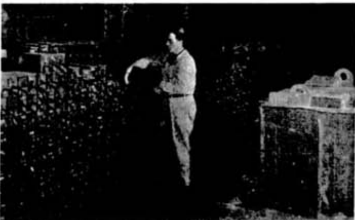
From the stockpile in the reverberatory department Nestor Mallette loads cans into a brick box which will be lifted by crane to the furnace of the roof under repair.
